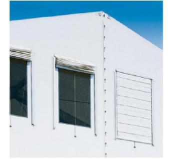
Cord-guided gable vent with folding cover (patented design), gable cover with plug fastening
